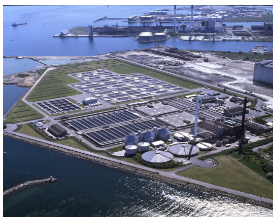
Figure 11.1. Negative impacts of nutrients, organic matter and industrial wastes on coastal waters, including seagrass beds, can be substantially reduced by treating waste water in advanced sewage treatment plants (with permission from Lynettefællesskabet I/S).
