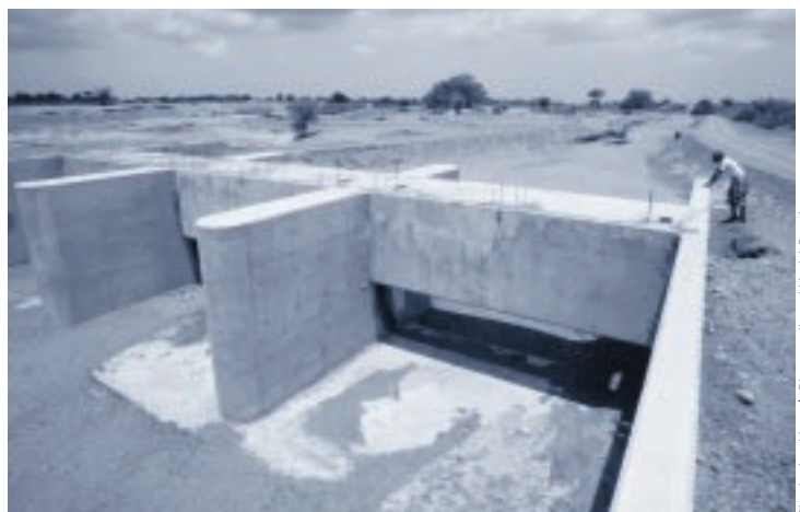
Weir under construction
