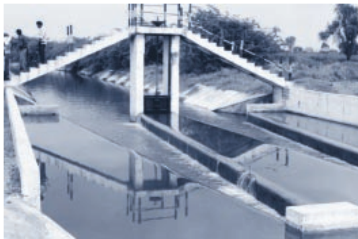
Long, crested weir regulator, Majalgaon, India
