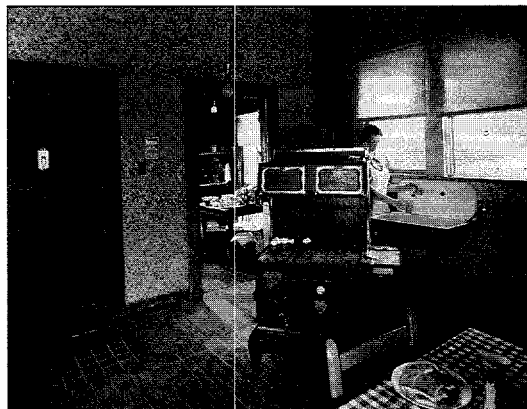
Rural home being electrified
