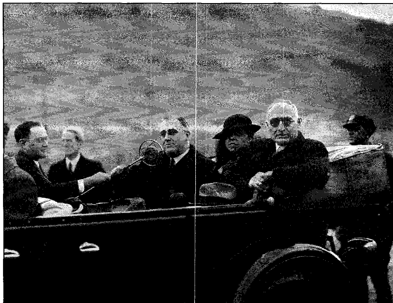
U.S. President Franklin Roosevelt, his wife, Eleanor, and A.E. Morgan at the Norris Dam construction site, September 1933
