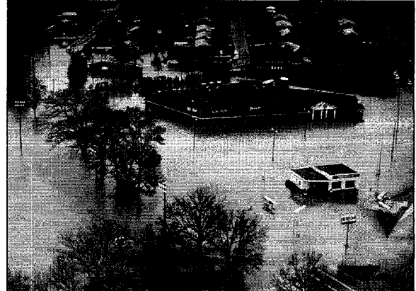
Flooding along the Tennessee River
