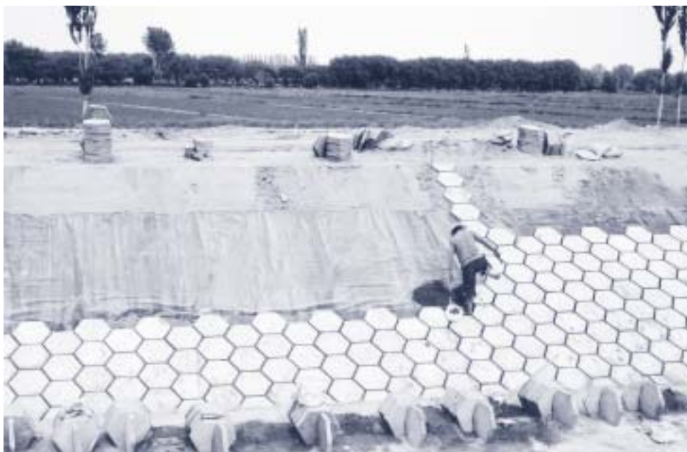
Canal lining with geomembranes, Tarim Basin, China
