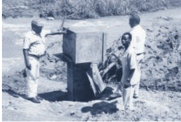
Siltation of gauging station, Pangani River, Tanzania
