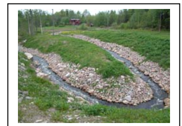
New fish by pass at the Finsjö hydropower station
